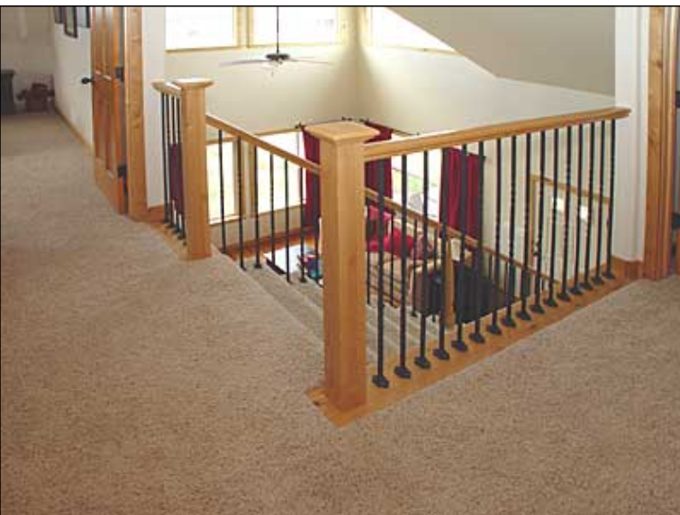
Iron spindled railing Ceiling fan
