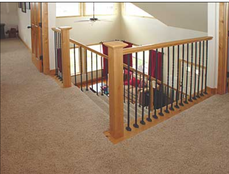
Iron spindled railing Ceiling fan
